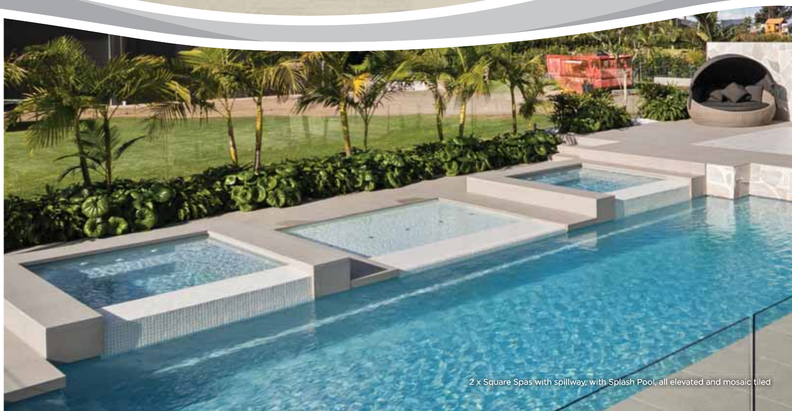
Elevated Square Spa with spillway and mosaic tiles
